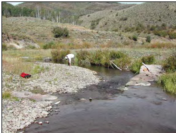
Figure 43: J-hook structure on the South Fork filling in by a point bar on the left bank opposite the tie-in ( 40^{\circ} 57.203' N, 107^{\circ} 05.163' W ).
