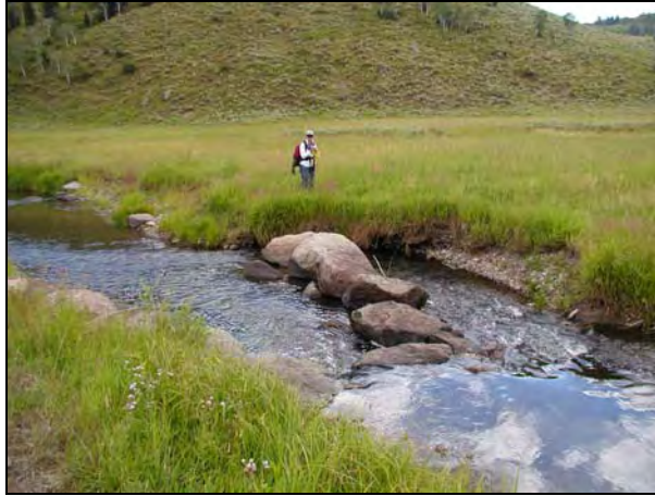
Figure 42: Photograph taken on August 23, 2005, showing a South Fork structure flanked on the right bank ( 40^{\circ} 58.327' N, 107^{\circ} 03.151' W ).
