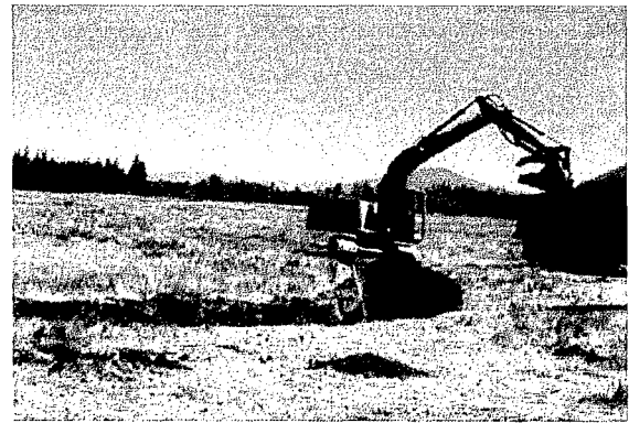
Figure 3 – Sculpting the restored channel in the summer of 1999 (Photos: Rick Poore).
