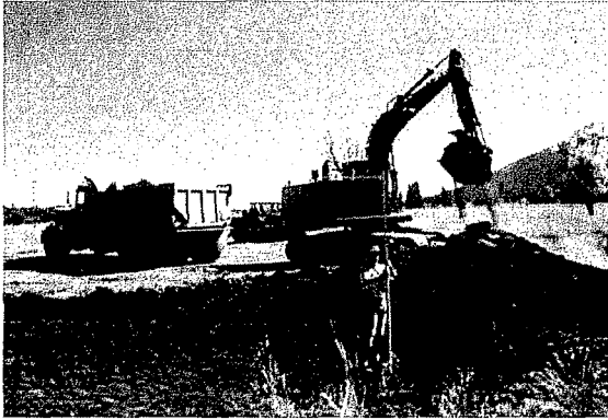
Figure 3 – Sculpting the restored channel in the summer of 1999 (Photos: Rick Poore).
